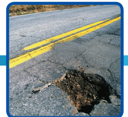
POTHOLES/DAMAGED PAVEMENT
